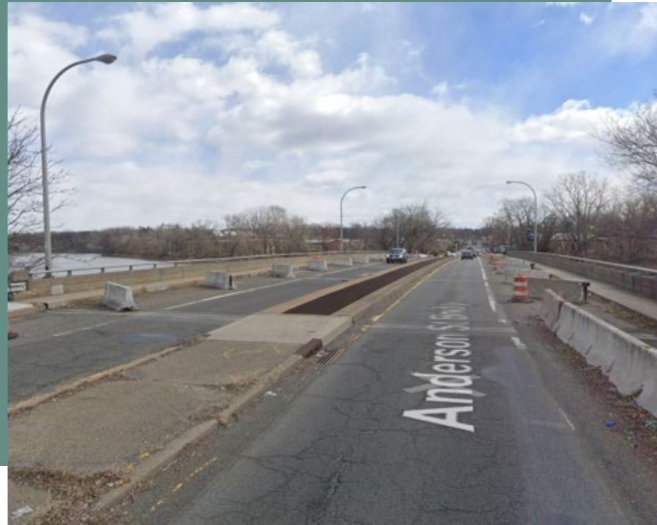
Anderson Street Bridge
