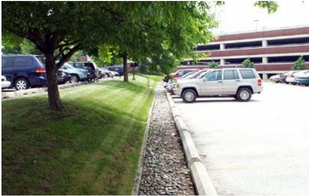
Infiltration beds in a parking lot
