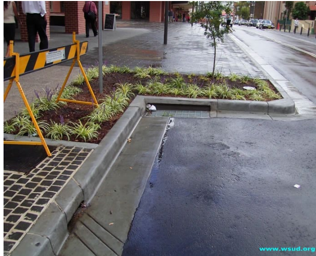
Street tree stormwater treatment retro-fit
