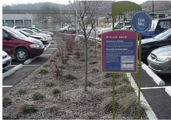
Bioretention swale in a parking area
