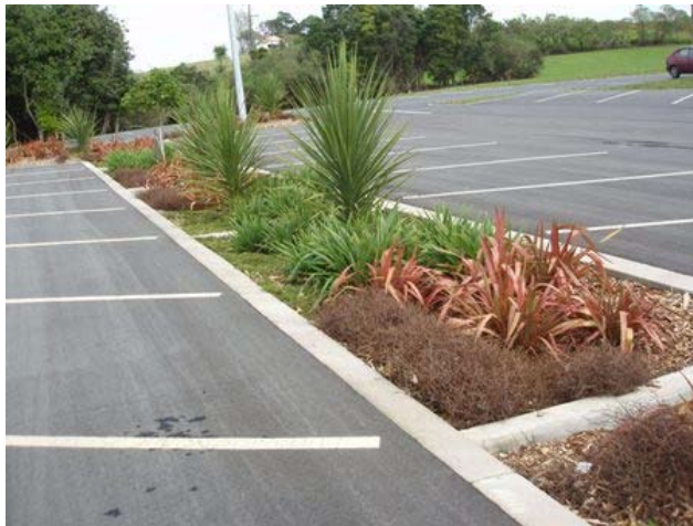
Rain Garden in Parking Lot
